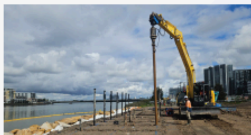
Recent works include seawall construction, screw piles and pathway progress
