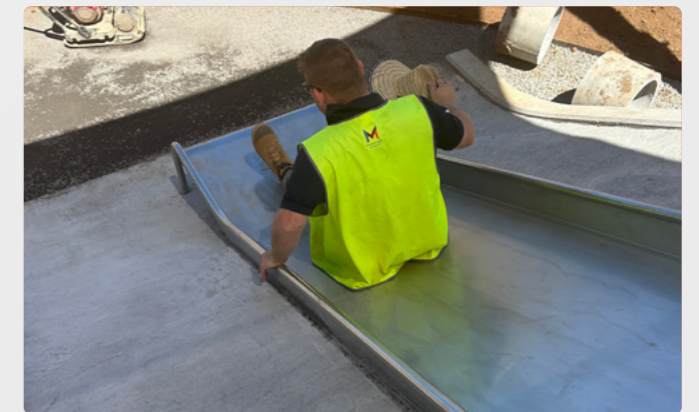
Important quality control testing on the new slide.
