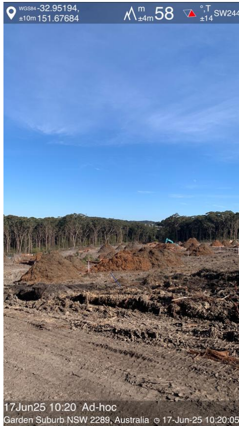
Figure 1-6 – Development footprint – earthworks
