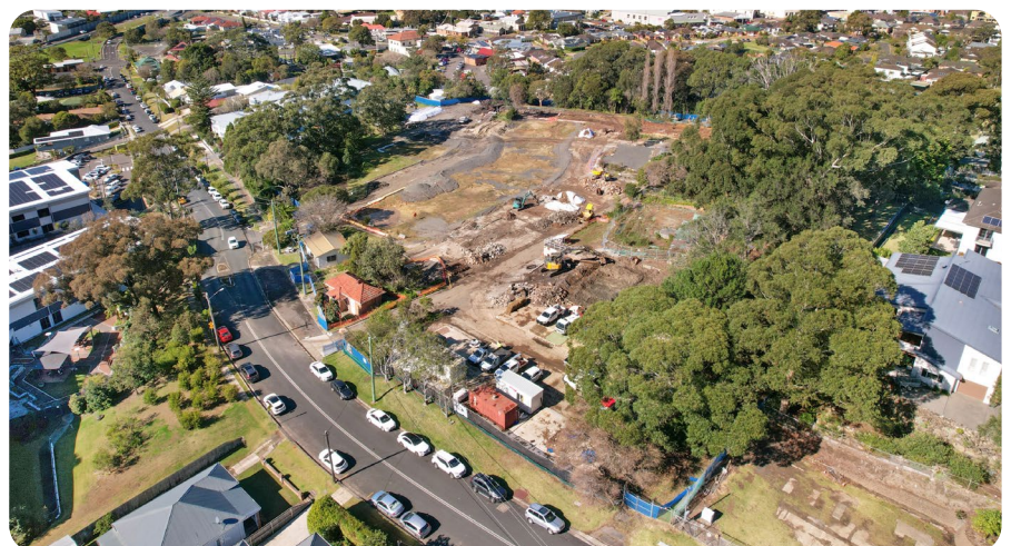
Bird's-eye view of progress
