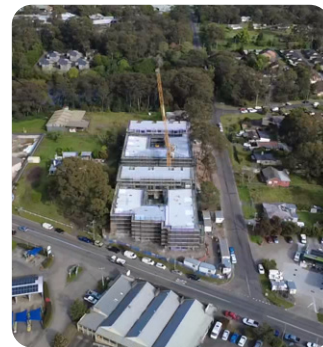
Roofing works complete on both buildings, ready for solar panels to be installed.
