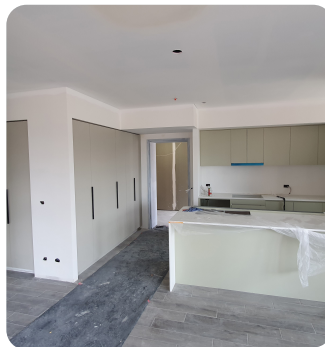
Kitchens taking shape, with benchtops and cabinetry being installed in the ground floor apartments.
