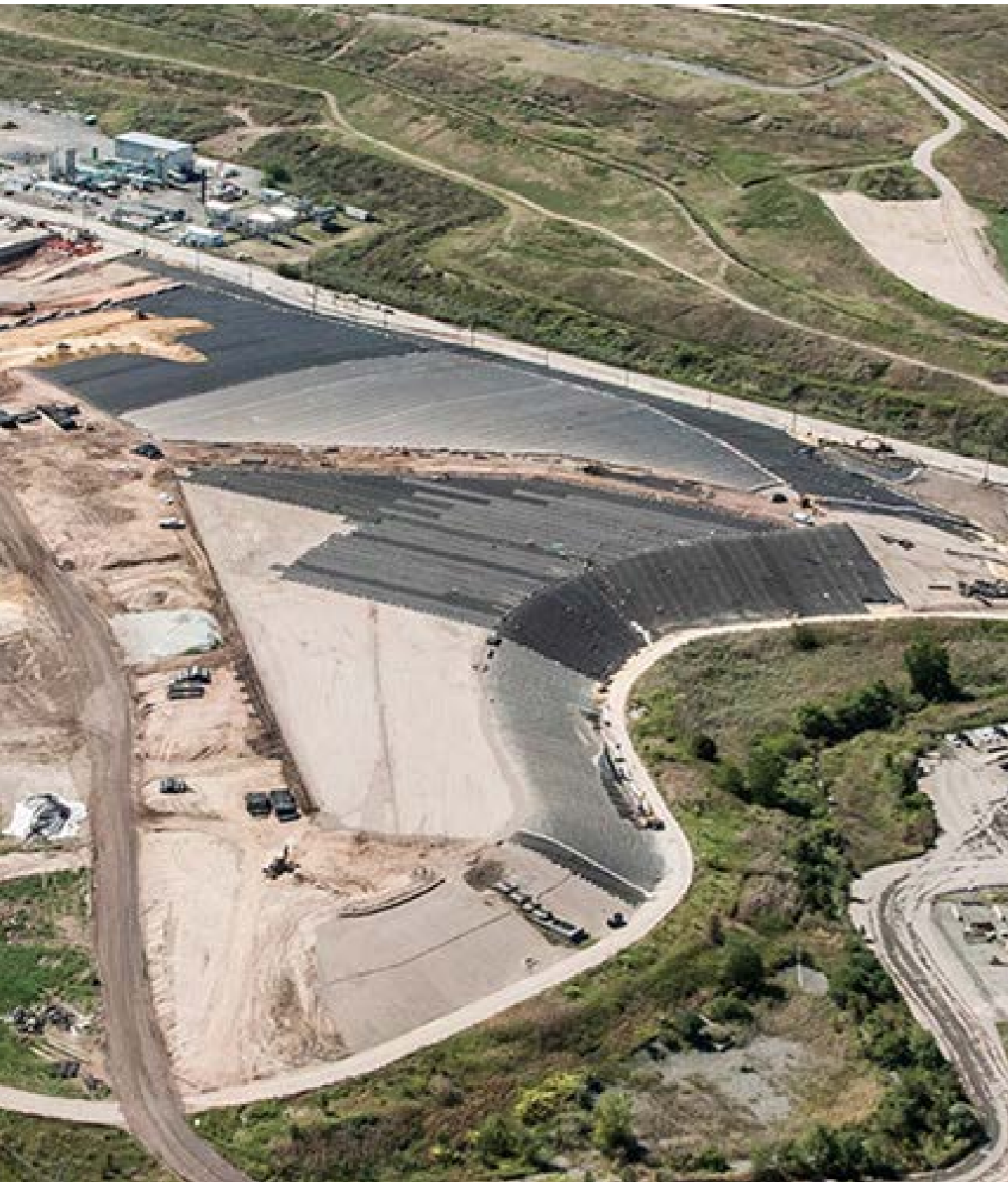
The process of capping 'Muldoon Avenue Mound' (completed in 2015) which relocated approx 305,822m 3 of waste. The cross section of the cap is made up of General fill, Select fill, two layers of geocomposite sandwiching a layer of geomembrane, barrier protection material, embankment fill, planting soil and seed mix with the erosion blanket. Image from Tully Construction, http://www.tullygroup.us/Capabilities/Environmental/Fresh-Kills-Landfill
