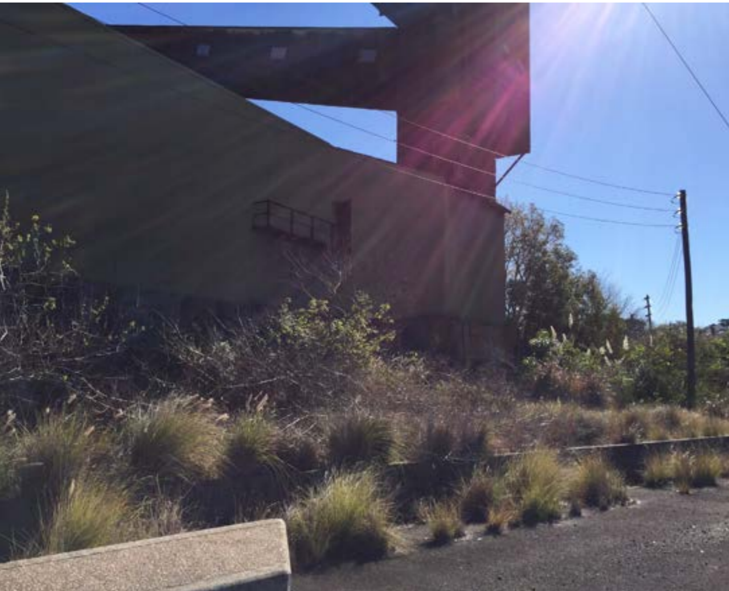
Looking north at the building toward the cooling ponds (Johnstone, 2017).
