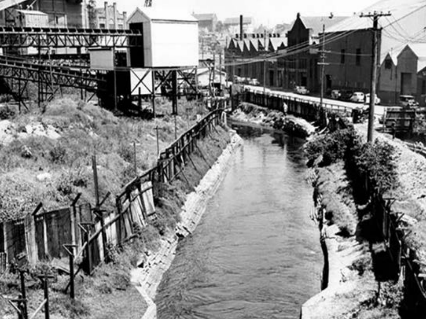
Cooling canal leading to the WBPS.
