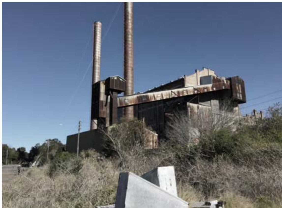
BEFORE: The location of Phytoremediation Garden 01 (Moulah, B, 2017).
