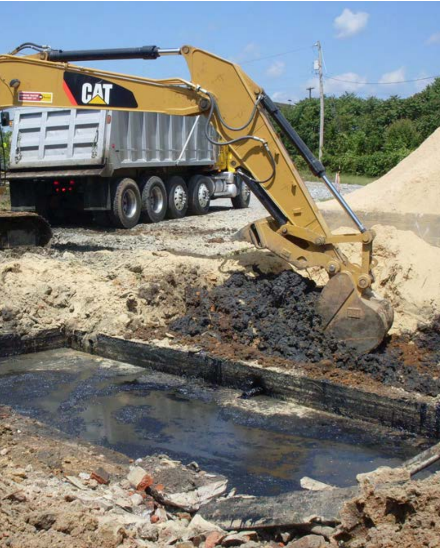
Example of soil contaminated with PAH's being extracted from a former manufactured gas plant in High Point NC. Image courtesy of NC DENR taken from ( https://sph.unc.edu/files/2014/10/High-point-qlg-004.jpg )
