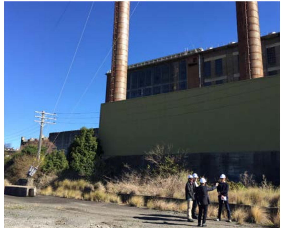
Looking south west at the building across the drainage channel and the Garden 1 site (Johnstone, 2017).
