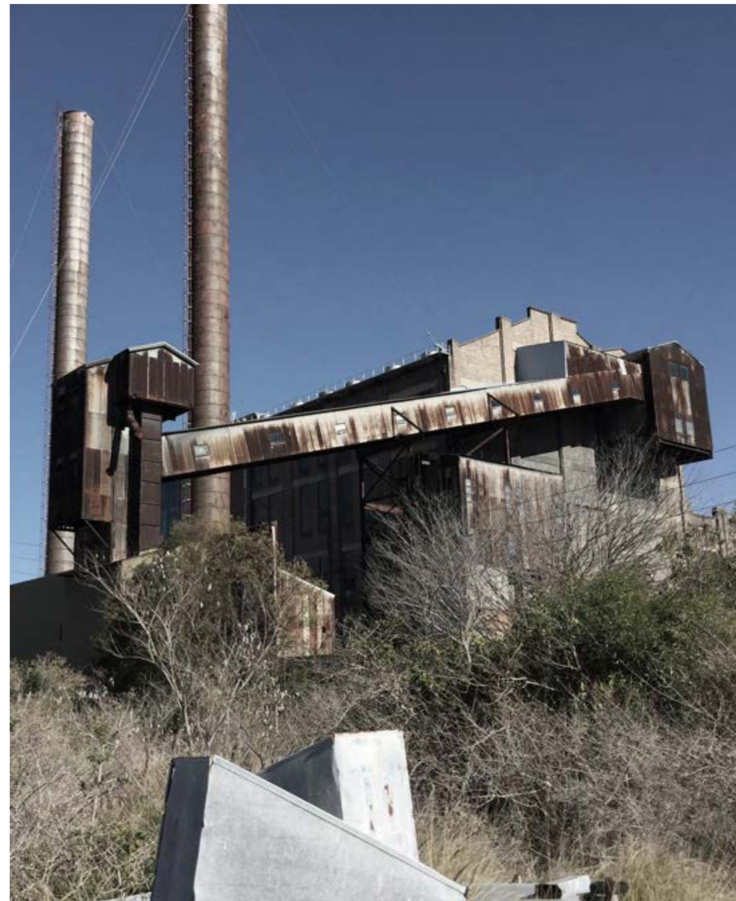
Photograph of specific site for Garden 01 with WBPS in the background (Moulah, B., 2017).
