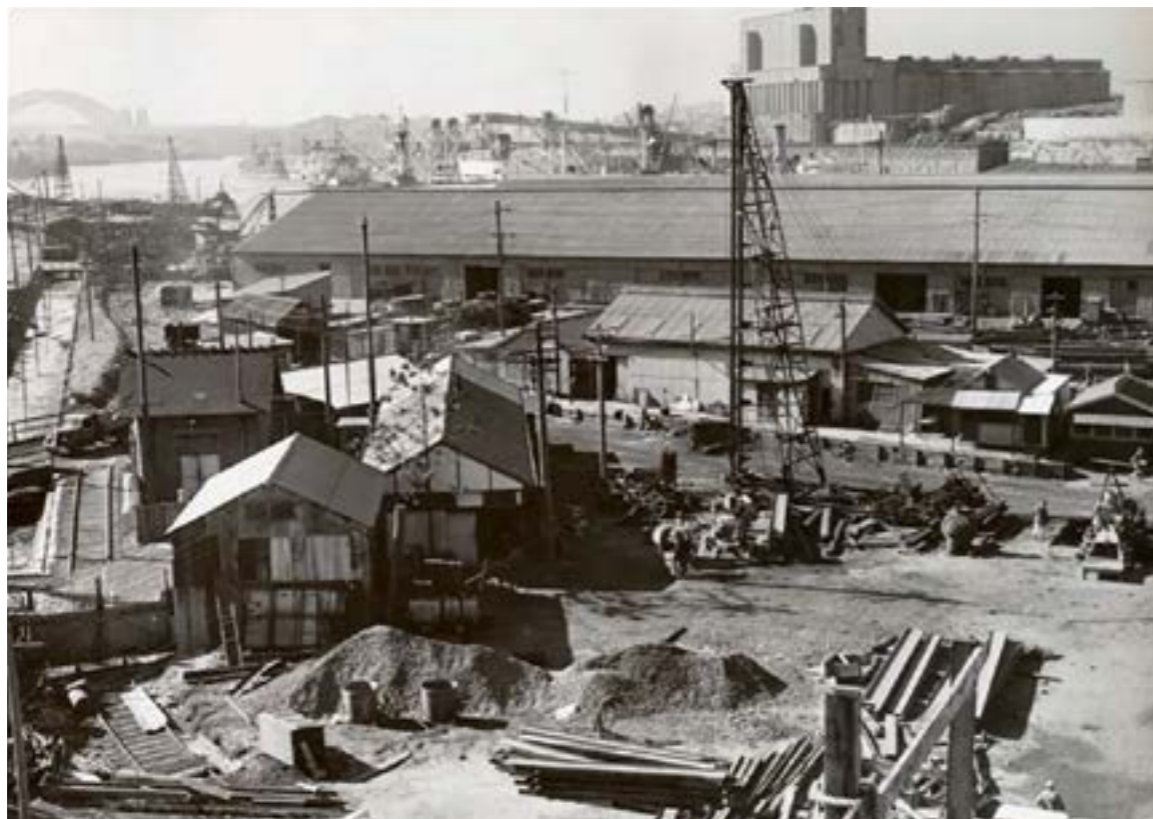
Material storage, WBPS.
