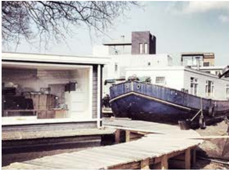
Site images taken during the construction of Park De Ceuveil (DEVLA Landscape Architects, 2014)
