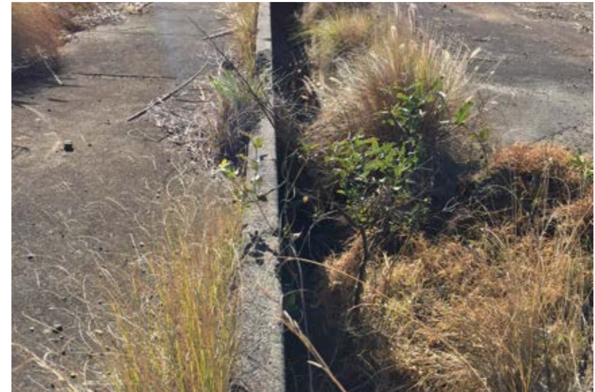
Looking north at the existing retaining wall and drainage channel which acts as the eastern barrier to the Garden 01 site (Johnstone, 2017).
