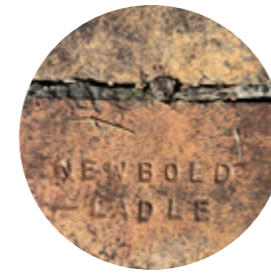
Ground Floor Walls Brick
