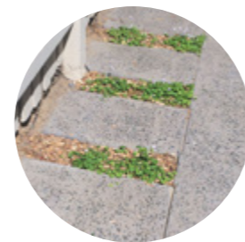
Concrete - Light or mid-grey colour with washed/exposed aggregate
