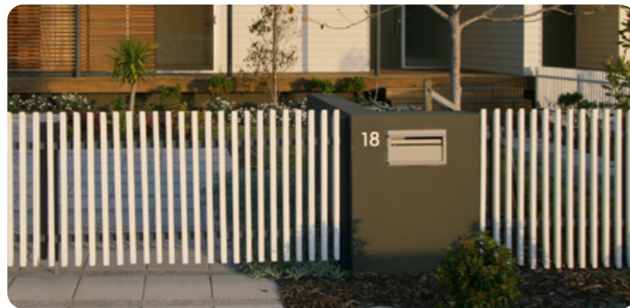
Fig 19. Contemporary interpretation of traditional picket fence - painted vertical timber slat front fence with mitred tops and bottoms, painted steel frame behind pickets in a dark colour to disappear into landscape. Masonry entry pillar with letterbox and street number.
