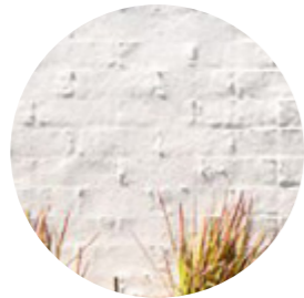
Bagged and painted brick
