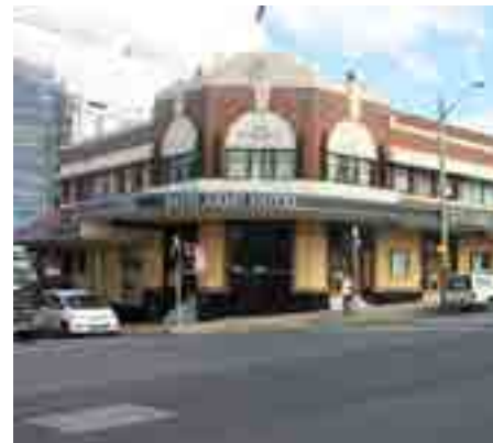
Figure 158. Burwood - existing hotel (Bath Arms)
