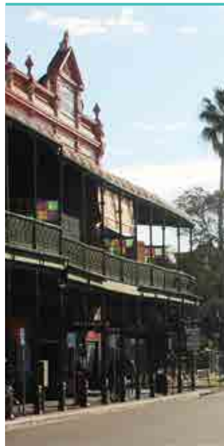
Figure 6. Facade detail, Johnston Street
