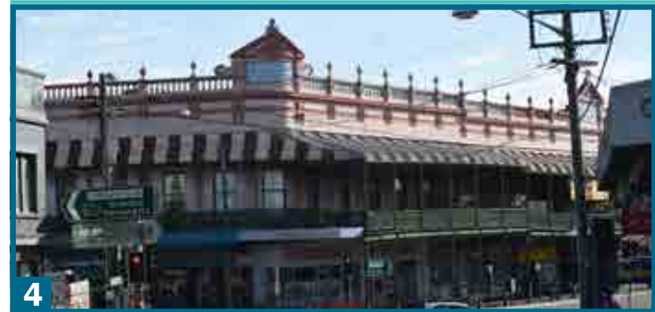
Figure 77. View of the Goodmans building on the corner of Johnston Street
