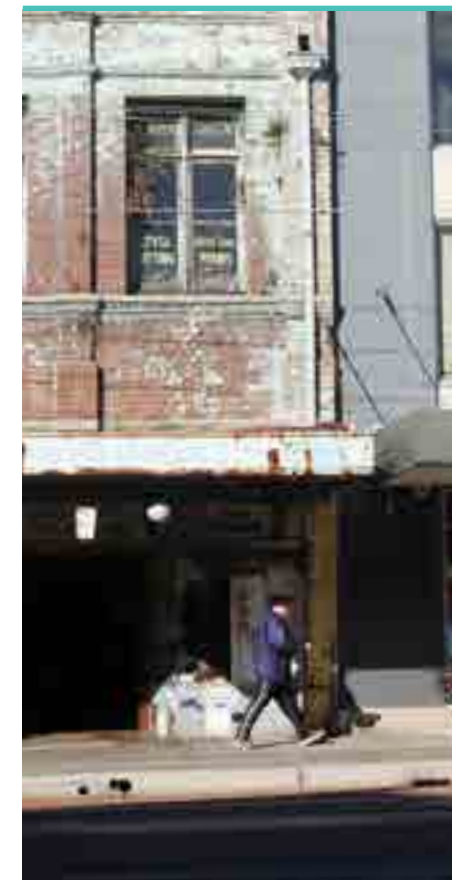
Figure 7. Facade detail, Parramatta Road
