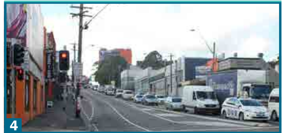
Figure 108. View looking west on Parramatta Road, to the Kennards Storage building
