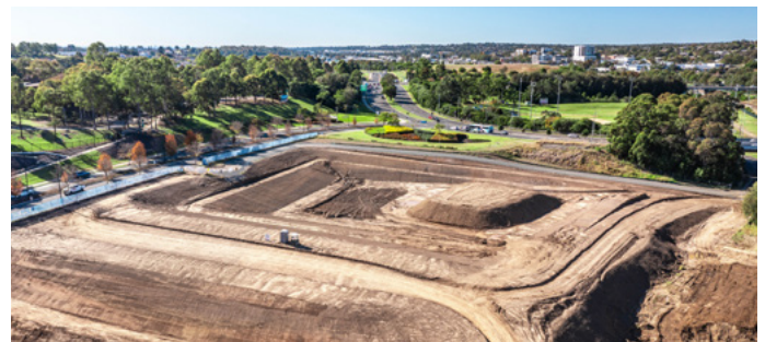
Macarthur Gardens North under construction
