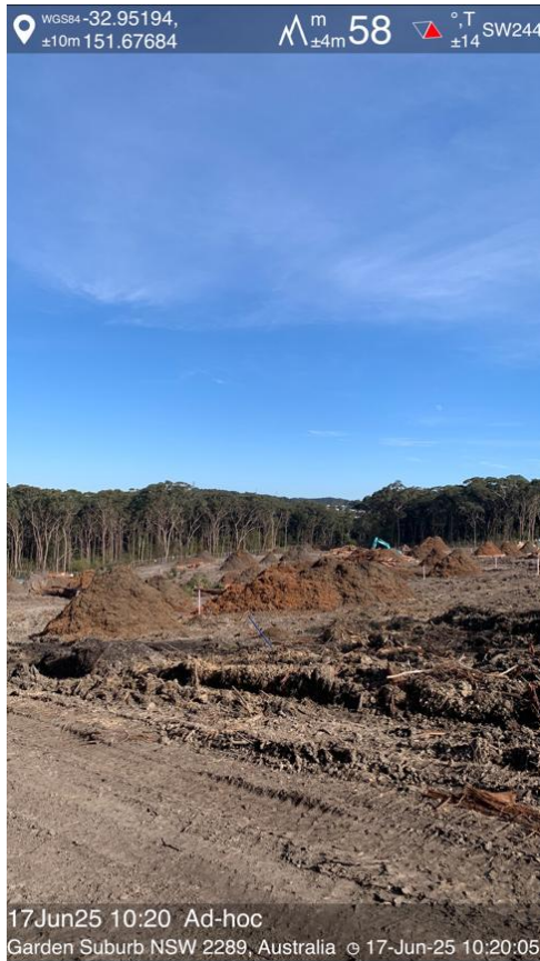
Figure 1-6 – Development footprint – earthworks
