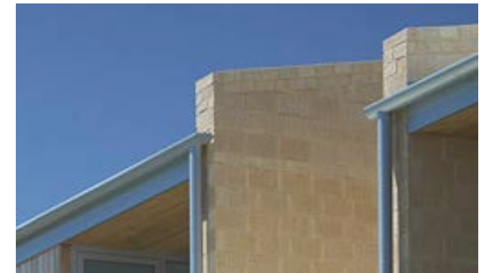
3 Designer block to party walls (Hope St Housing. OW and MDC Architects)
