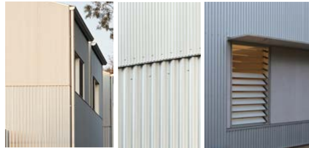
2 Varying scales of metal cladding profiles (Maggie Street Curious Practice. Image Alex McIntyre)
