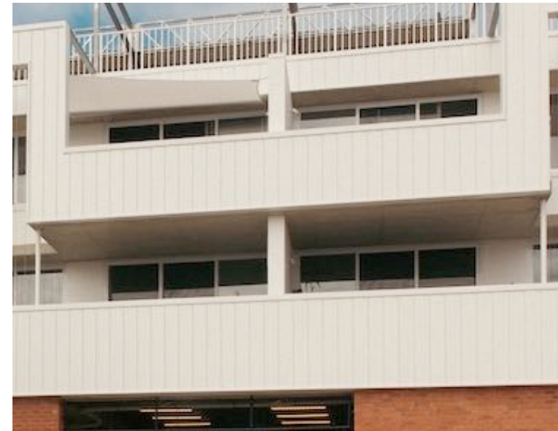
1 Metal cladding to dominant wall plane and balconies (Nightingale Fremantle. Image Kate Longley)
