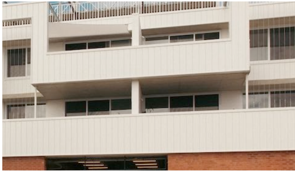
1 Metal cladding to dominant wall plane and balconies (Nightingale Fremantle. Image Kate Longley)
