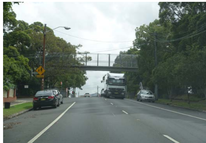
Figure 2.8: Existing condition (Taverners Hill)
