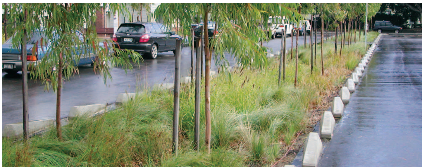
This street has a swale within its central median as part of the WSUD strategy. The unique kerb treatment and timber walkway also create an interesting streetscape.
