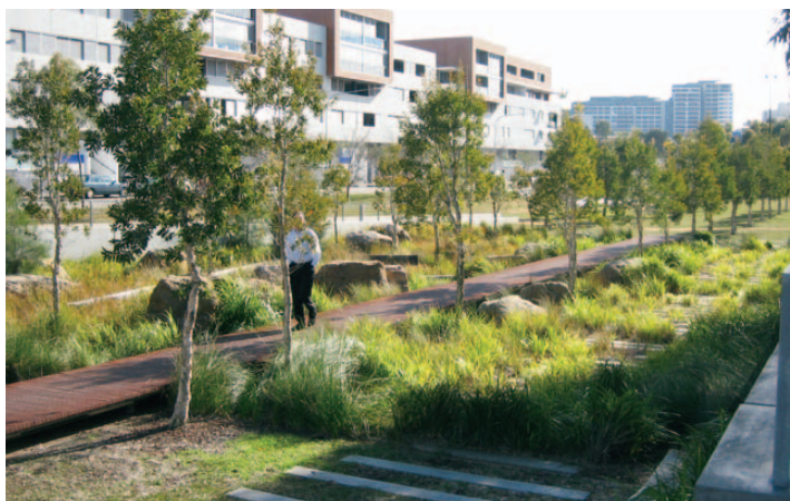
Vegetated swales: are constructed vegetated depressions that collect and direct stormwater runoff from impervious hard surfaces such as roadways, car parks and paving to areas that will benefit from irrigation. Photo – Vegetated swales, Victoria Park
