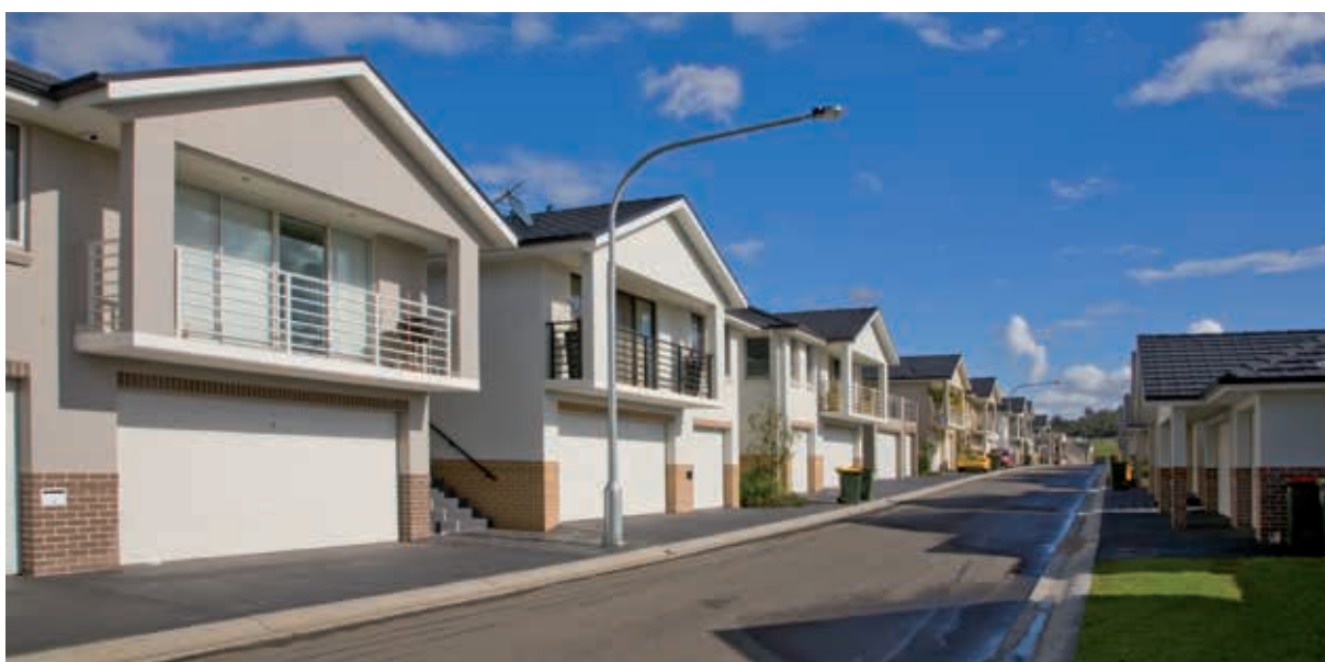
Garage-top studios | Garden Gates, Mt Annan
