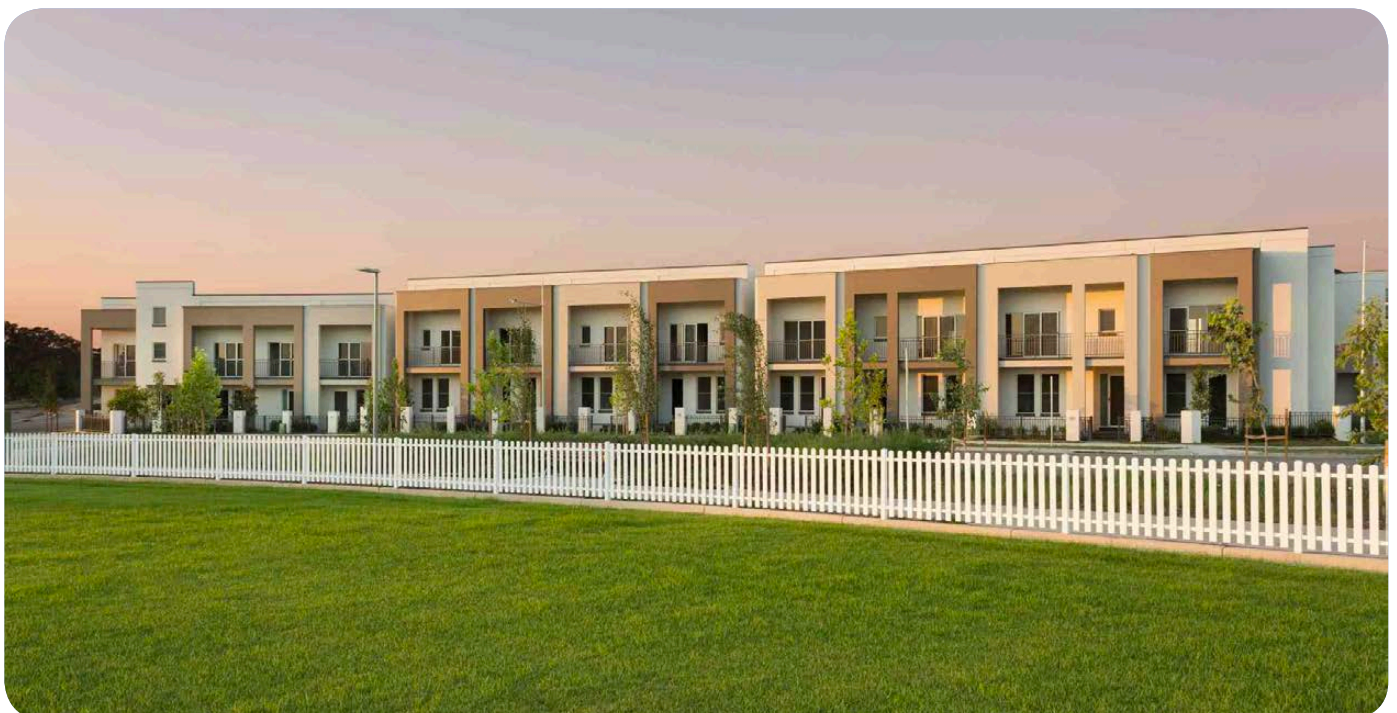
21st Century Housing, Thornton
