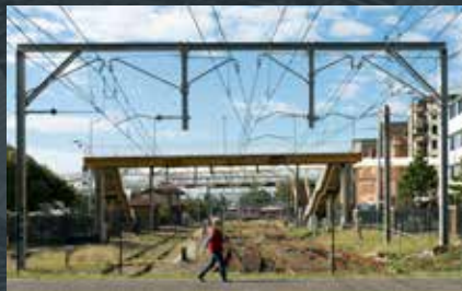
Rail Corridor, Newcastle.
