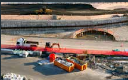
Construction works, Green Square.
