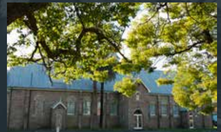
Recreation Hall, Parramatta North.
