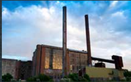
White Bay Power Station.
