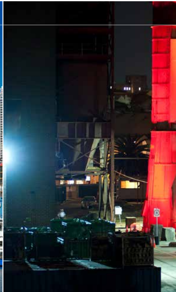
White Bay Power Station.
