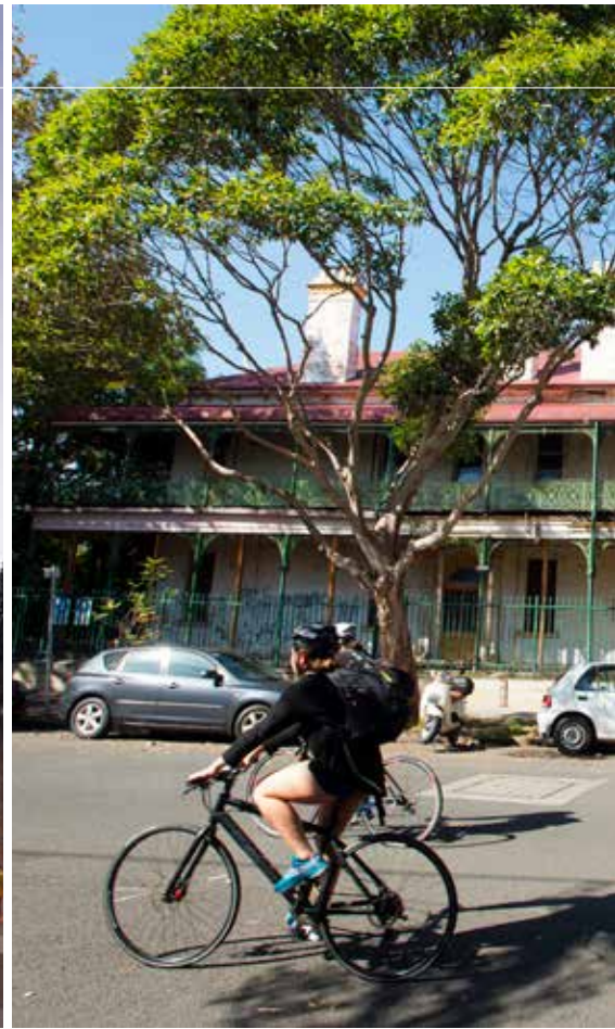
Heritage listed Chief Mechanical Engineer's office, Central to Eveleigh.
