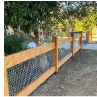
Lots facing biodiversity conservation area must have dog proof front fencing. For example mesh alongside post and rail.
