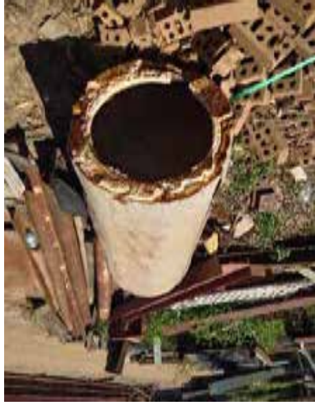
Photograph 42: Potential ACM pipe on Parcel 7
