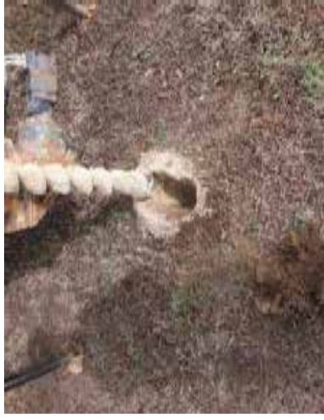
Photograph 72: Geotechnical bore drilled on Parcel 16. Shale shown
