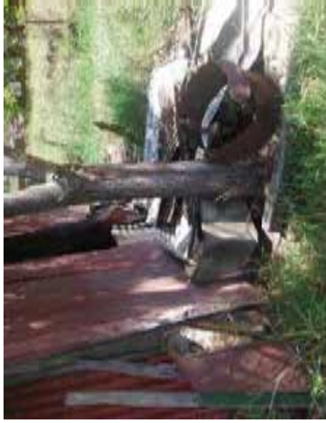
Photograph 122: Building materials on Parcel 28
