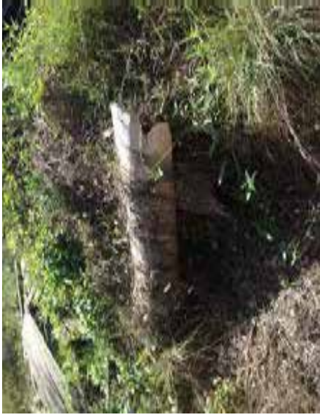
Photograph 164: Potential ACM on Parcel 42
