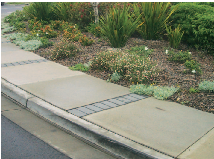
The simple use of inset pavers within the footpath can add interest and help to tie in grey driveways through the estate as part of a coordinated approach.
