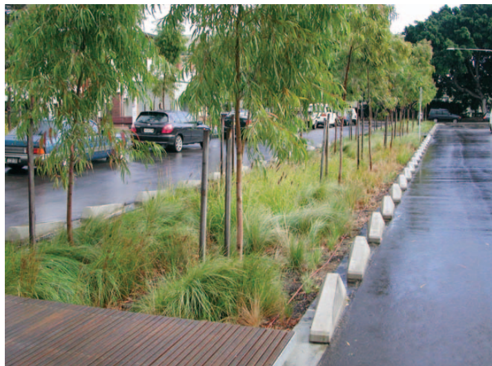
This street has a swale within its central median as part of the WSUD strategy. The unique kerb treatment and timber walkway also create an interesting streetscape.
