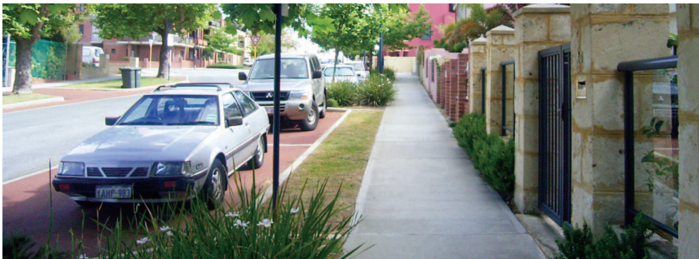
The verge in this street is well defined with a strong alignment created by the fence, the simple footpath, grass verge and rain garden with street trees. It creates a pleasant ambiance for pedestrians. Generally the parking bay would not be a different colour to the roadway as in this image and the cycleway would be combined with one of the street footpaths for safety.
