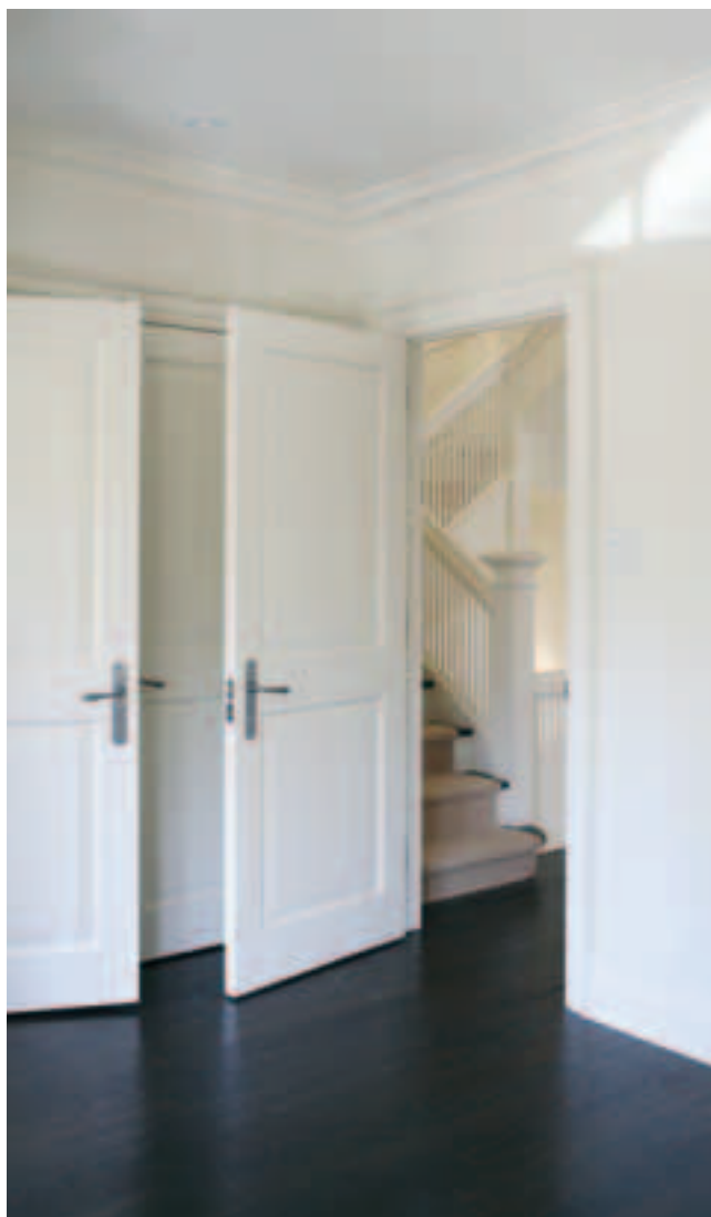
An 820mm clear opening generally requires an 870mm door leaf.
