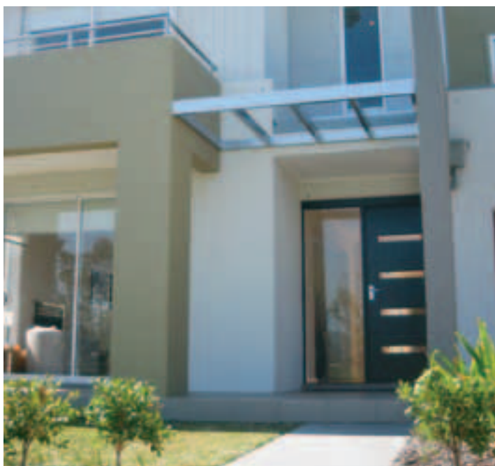
In this example, the window panel next to the front door improves perceived security, as the resident can see who is on the other side.
