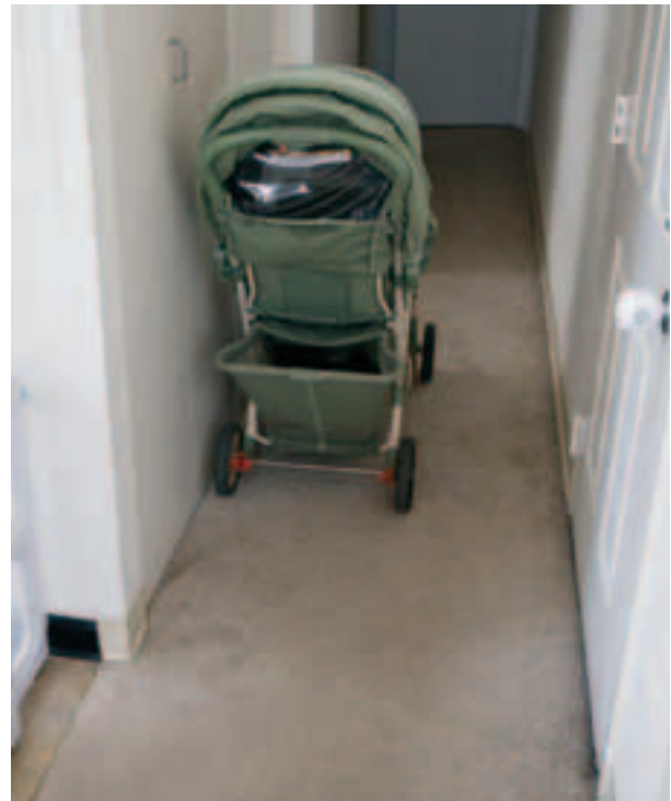
Tight corridors leave little room for 'living'.
