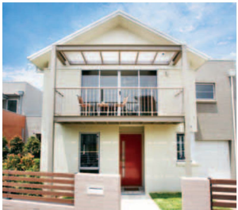
A level path from the footpath to the front door makes access easier.
