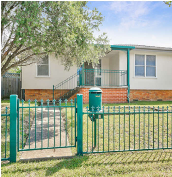
Example of a cottage, refurbished and sold by Landcom.
