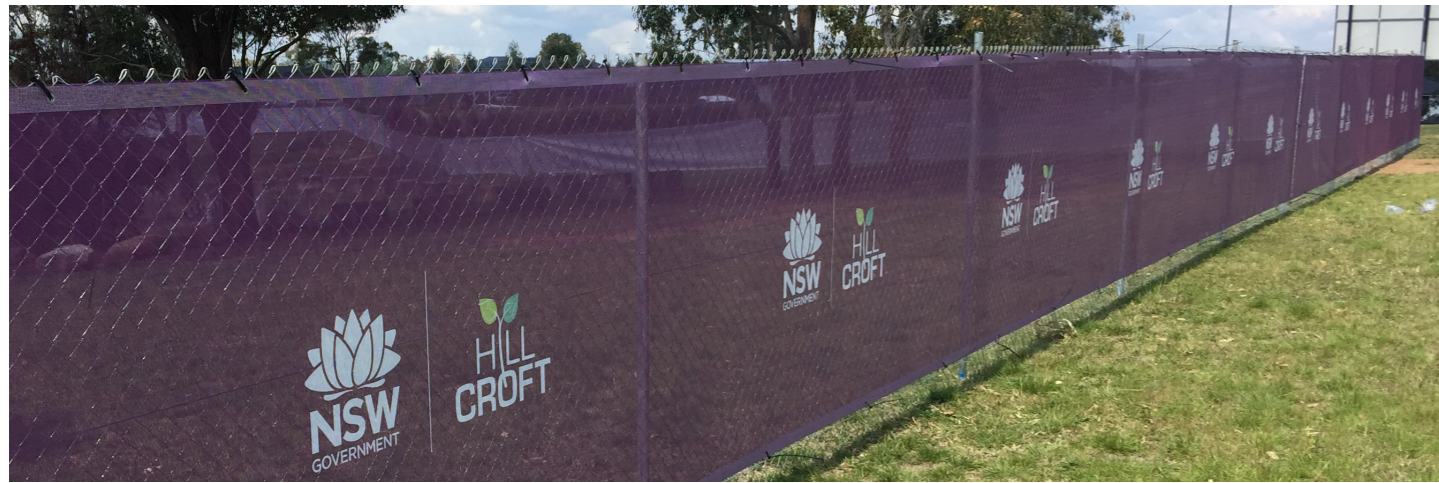
Early works are underway on Stage 3
