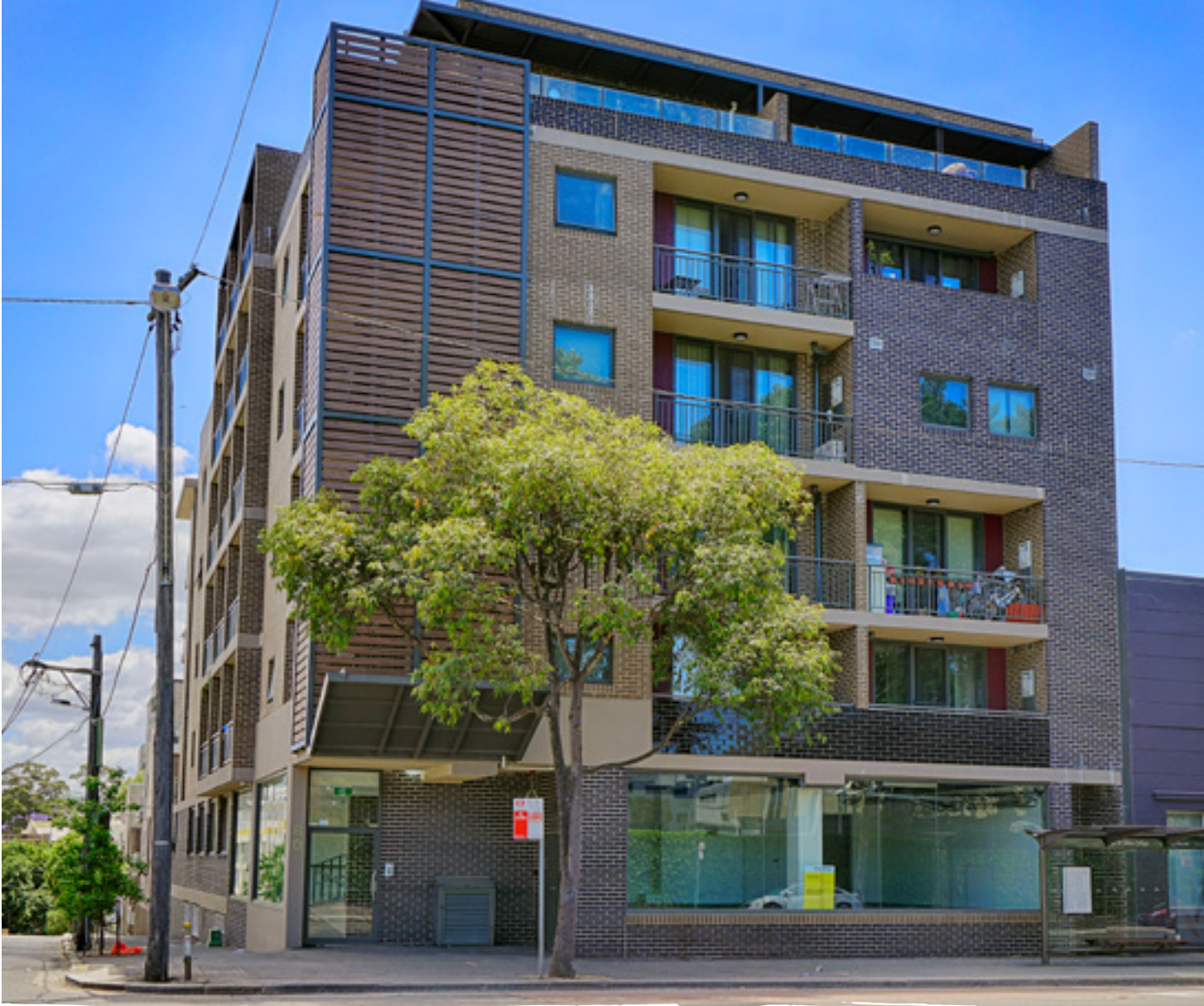
Boyce Group - New Generation Boarding House, Camperdown, Sydney
