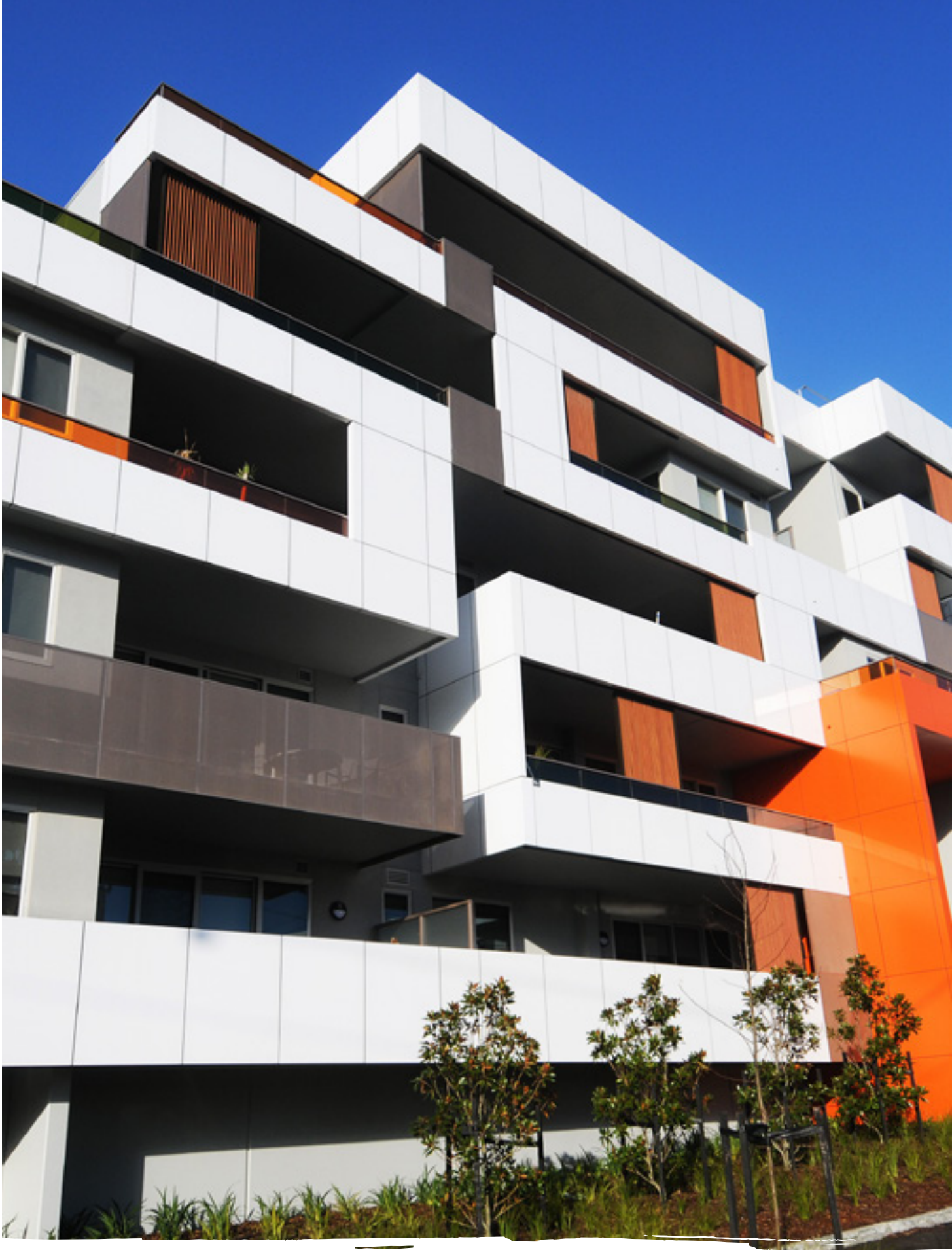
Port Phillip Housing Association (now Housing First), Ashwood, Melbourne - affordable rental housing
