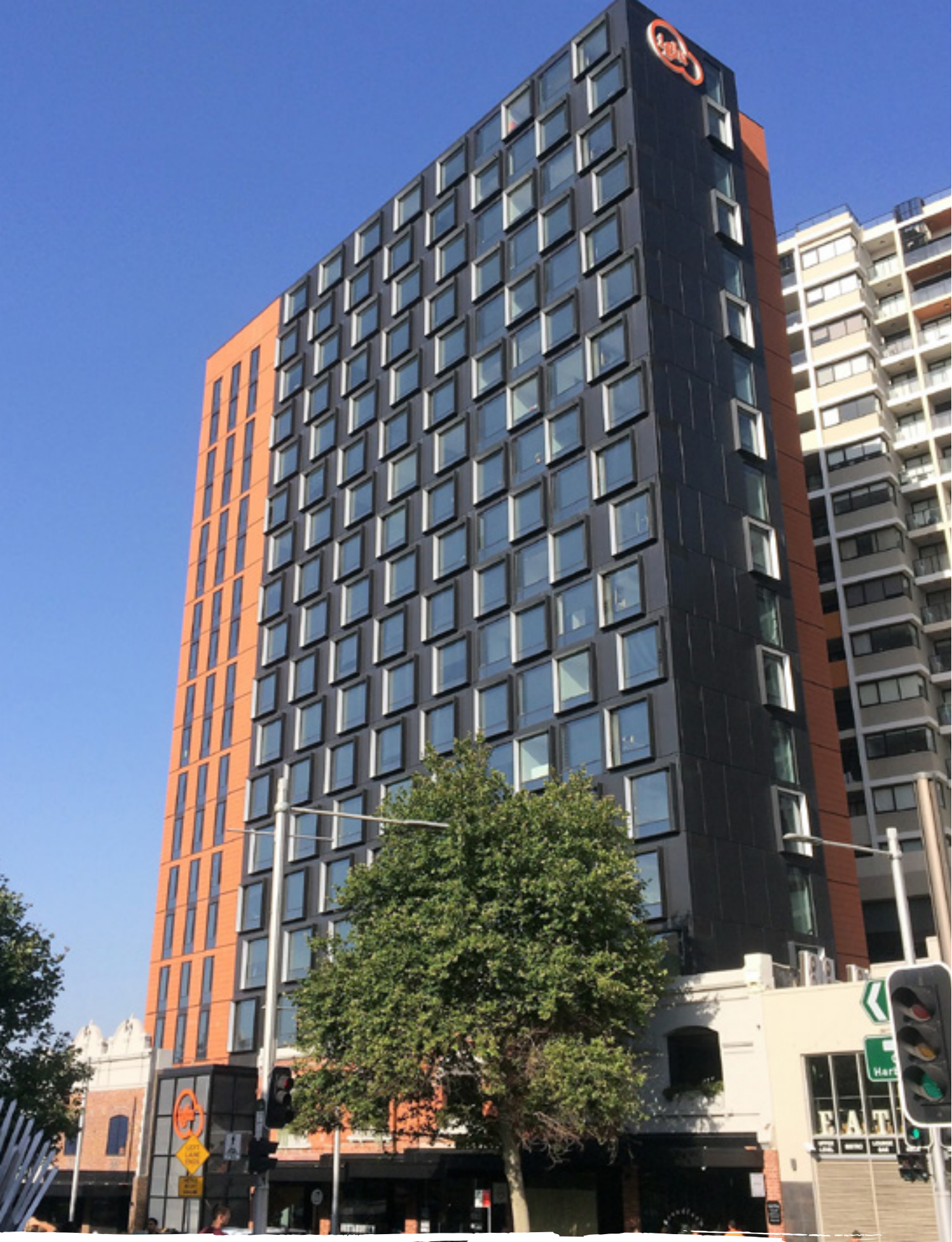
Iglu - purpose-built student housing - Redfern, Sydney
