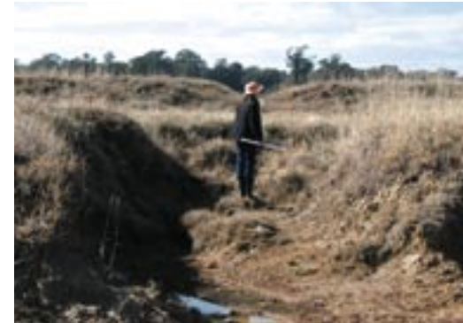
Bank erosion of watercourse has led to the exposure of the B-horizon sodic soil.
